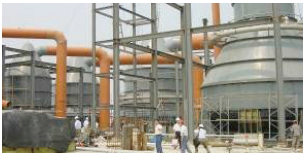
Installation of NaCl/Na 2 SO 4 combined plant
