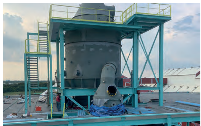
MVR crystallizer under construction
