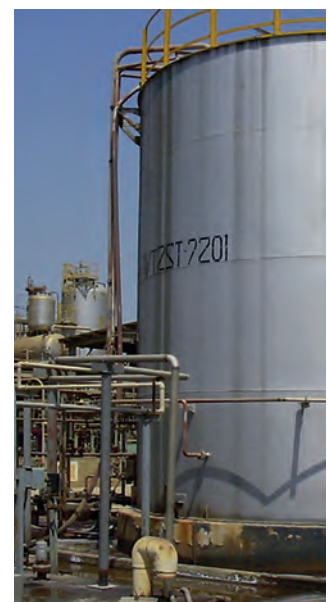
Waste Water Pretreatment Tank
