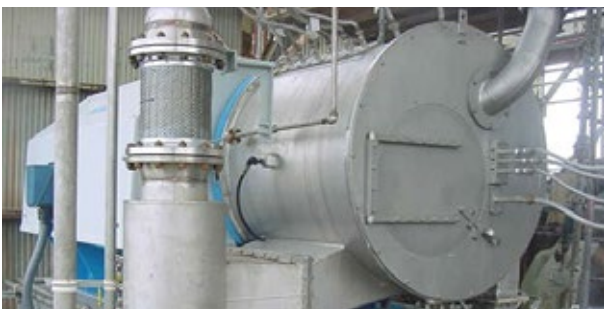
Pusher-type Centrifuge
