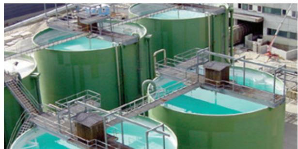
Brine Purification Plant
